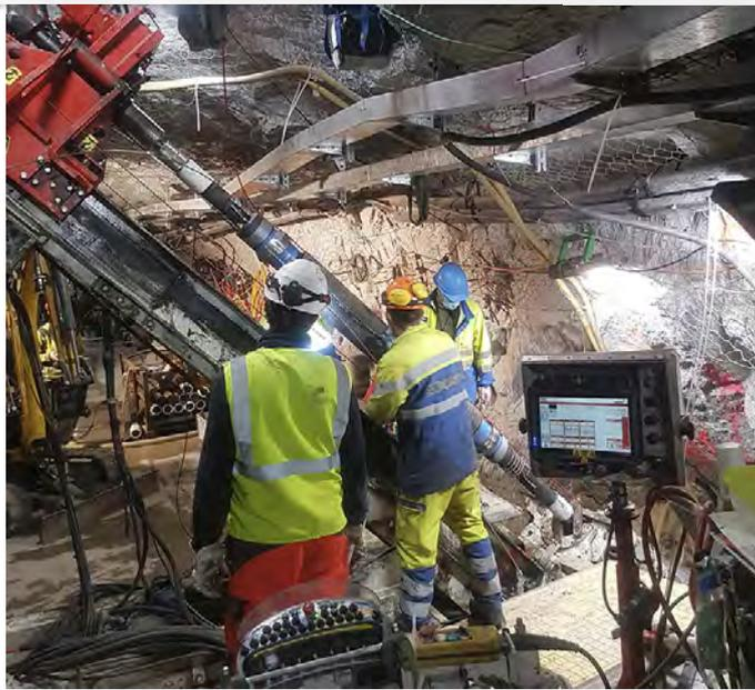
Image: The first packer during installation. © Swiss Seismological Service at ETH Zurich, 2021.
