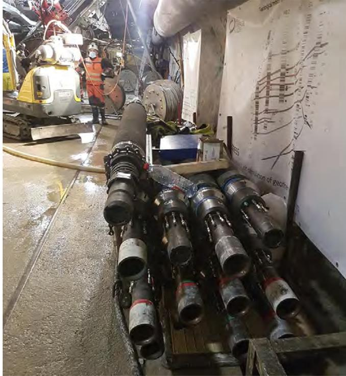
Image: All the multi-packers, ready to be installed in the borehole. © Swiss Seismological Service at ETH Zurich, 2021.
